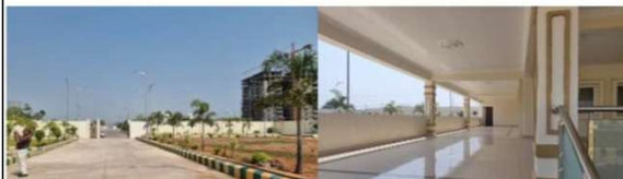
Integrated Township, Nalgonda, Telangana
