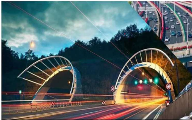
Bengaluru Twin Tunnel Corridor Project
